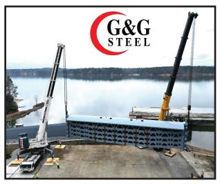
**G&G STEEL.** A joint project of the Russellville and luka facilities, G&G Steel delivered the first of two lift gates to a lock and dam near St. Louis. The lift gates were fitted, welded, painted, assembled and loaded on barge at Tri-State Commerce Park. The gates are 110 feet long and weigh 520,000 pounds each.
