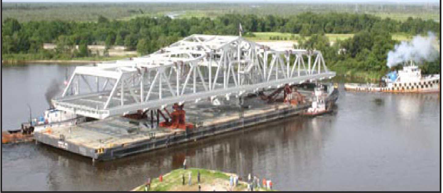
Shown above is a bridge fabricated by G&G Steel and featured on the Discovery Channel.
